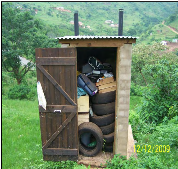
Plate 6.4: Use of UDD Toilets as a Storeroom
