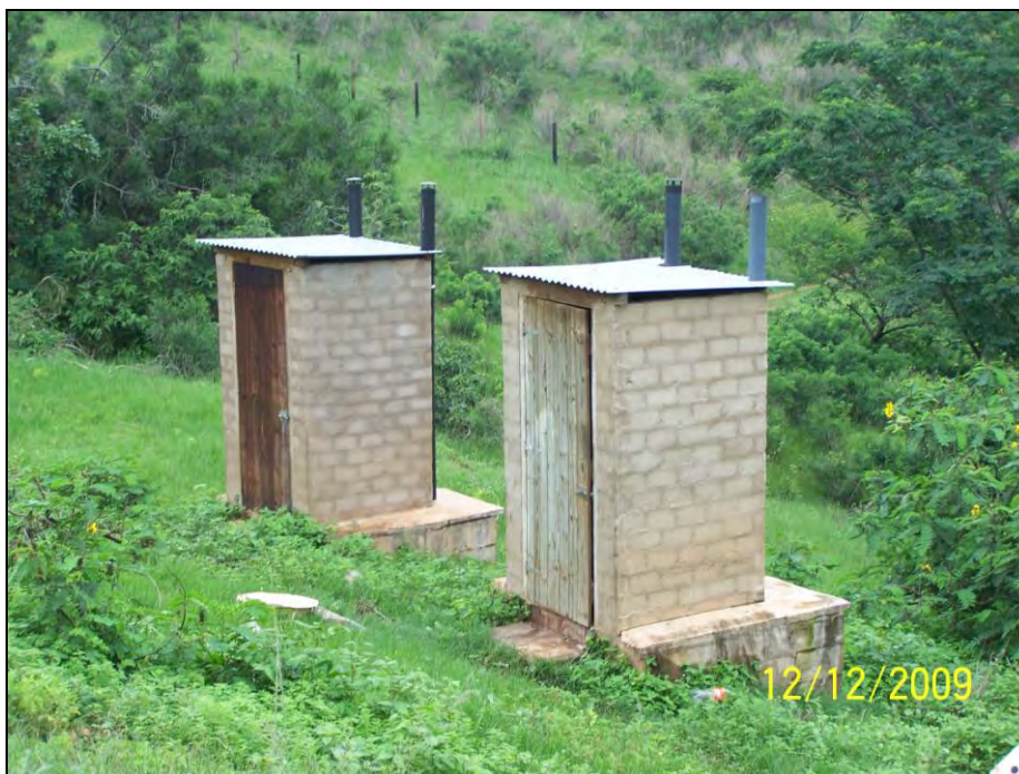
Plate 6.3: Rural Toilets constructed too far from House
