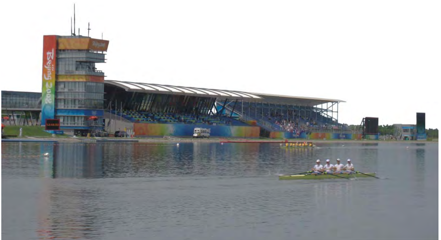
Illustration 04.34: The Finish Tower (left), Spectator/Grandstand building (middle), temporary spectator grandstand (right) and video boards (far right)
