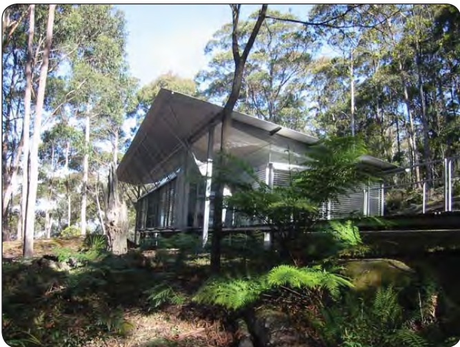
Illustration 03.06: Simpson-Lee House , by Glenn Murcutt, which nestles into its natural surroundings. Source: www.archnewsnow.com
