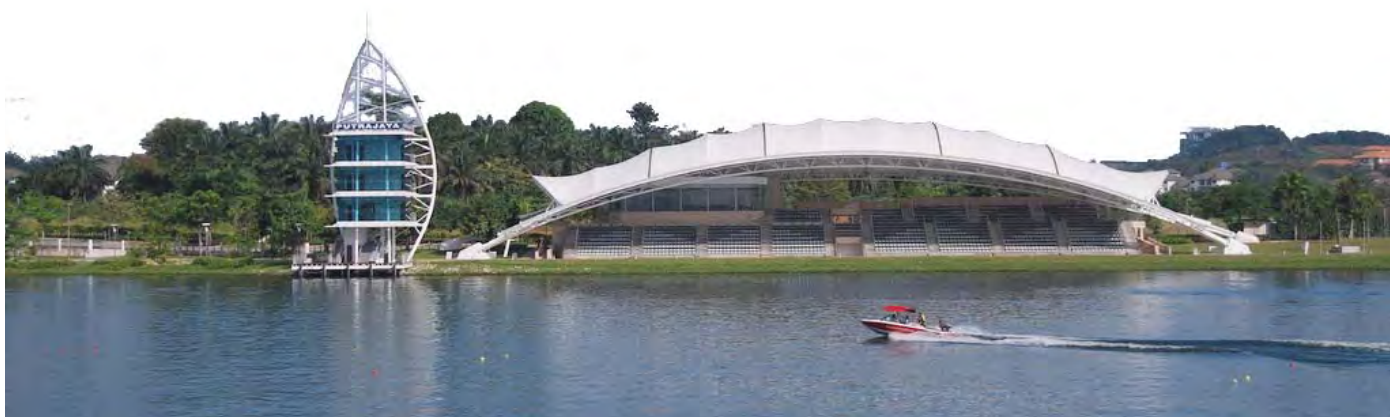
Illustration 03.02: The Putrajaya Water Sports Centre in Malaysia.
