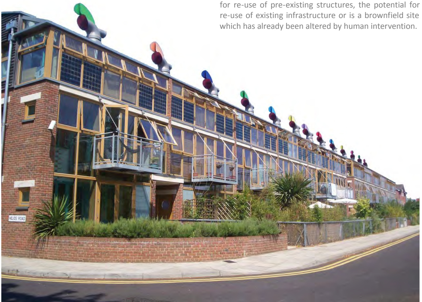
Illustration 03.14: The Beddington Zero Energy Development (BedZED) in England by Bill Dunster, is built on reclaimed brownfield land. Source: www.flickr.com
