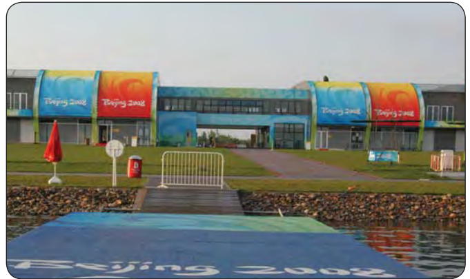
Illustration 04.46 The walkway connecting the two buildings. Source: BlighVollerNield Architects
