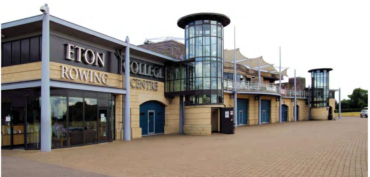
Illustration 04.59: Front view of the main building at the rowing centre.
