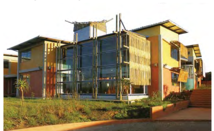
Illustration 03.13: The Africa Centre, by East Coast Architects which successfully used local labour and materials in its construction.
