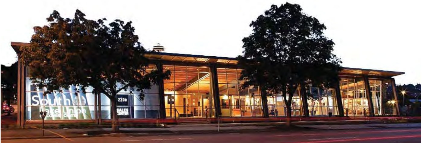
Illustration 03.22: Seattle's 'Pavilion in the Park', designed by Miller|Hull Architects, displays a 'cradle-to-cradle' nature as it can be completely disassembled and transported to a whole new location by breaking it into four separate modules. Furthermore, the building can be expanded or reduced as needed. All the materials of the building are environmentally-responsible materials, putting emphasis on recycled content and durability.
