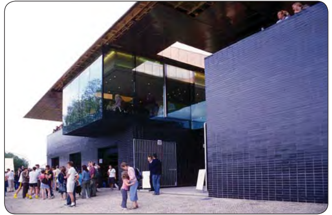
Illustration 04.07: The front of the boathouse, with glass 'club room' projecting out towards the river.
