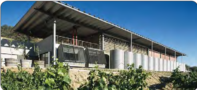
Illustration 03.18: A winery in Australia by Glenn Murcutt boldly expresses rain water tanks as part of the buildings facade.
