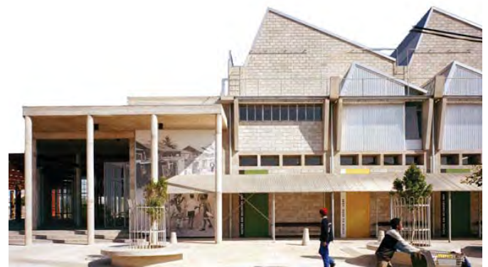
Illustration 03.11: The Red Location Museum in Port Elizabeth by Noero Wolff Architects uses low/tech maximum-benefit solutions in its construction. Materials such as standard steel windows, concrete blocks, and gum poles are used in unconventional ways to great effect.
