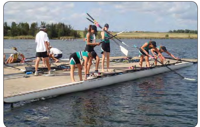
Illustration 07.21: One of the launching pontoons at the Sydney International Regatta Centre.
