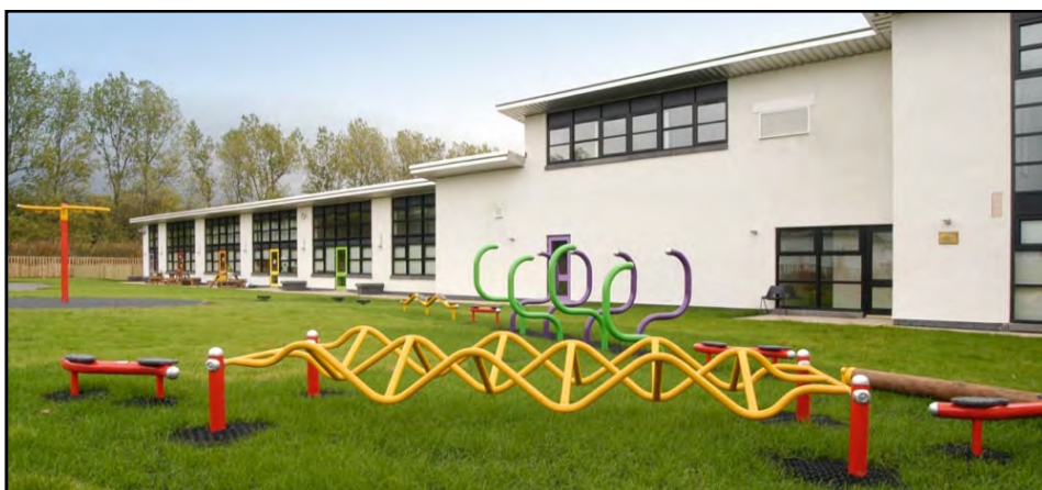
Figure 5-7 Play Equipment in the Outdoor Area (Courtesy of Aitken and Turnbull Architects)
