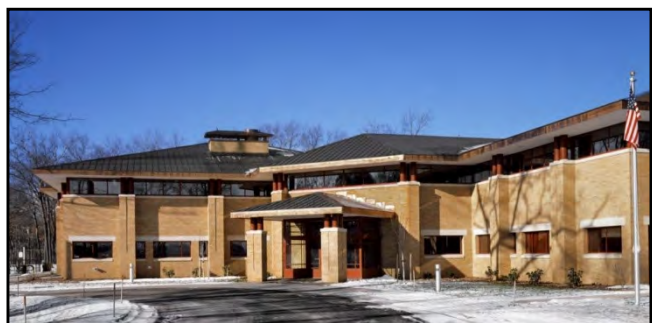
Figure 4-12 Large Overhangs at River Street School, Windsor, by James Vance and Associates, Eliminates Contrast and Glare (Henry, 2011)
