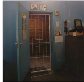
Figure 6-14 Security Gate on a Classroom Door
