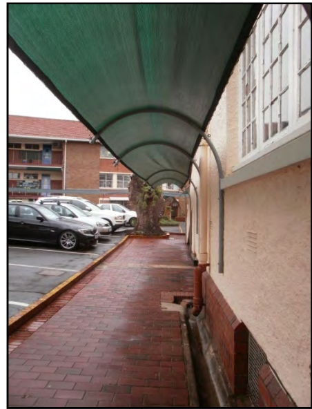
Figure 6-19 External Walkways with Cloth Roof Structures
