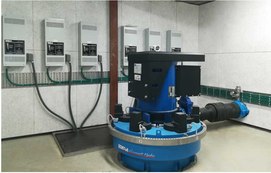
Figure 2.10: Typical installation of a hydraulic group
