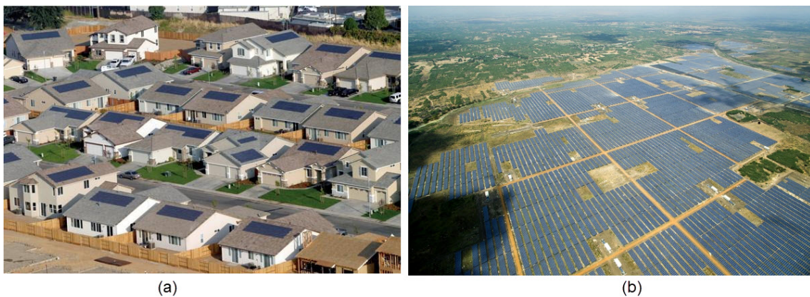
Figure 2.4: (a) Little distributed solar generators. (b) Solar Plant
