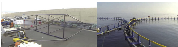
Fig. 6. Left, the S3 floating structure on the quay of the port ready to be transported to the cages. Right, surface view of its position between two cages during transfers.
