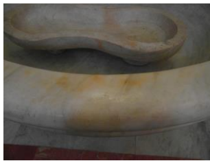
Efflorescence (e)
