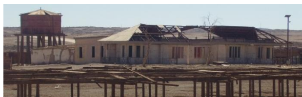
Chalet del Inspector General, 2008
