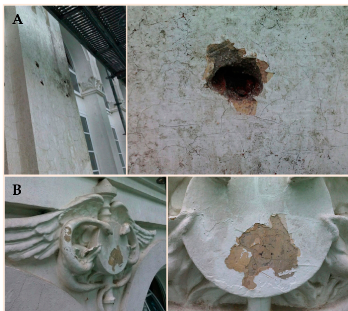
Figure 2. General image (left) and detail (right) of the sampled areas of the building: (A) pillar and (B) ornamental part. Photographs: Marta Díaz.
