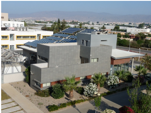
(a) Overview of the building
