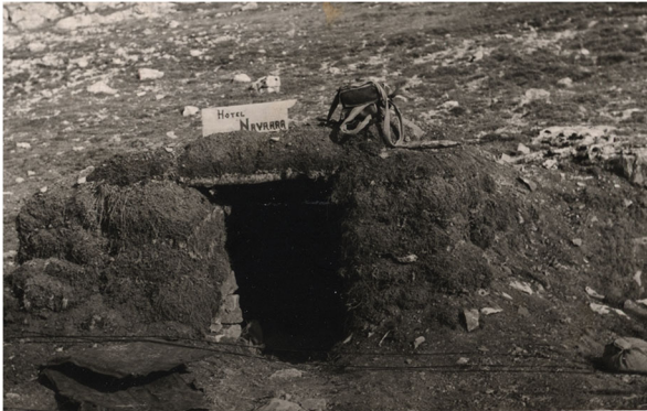
Fig. 4. Photograph from 1937 showing a small shelter built of stone and wood and covered with turf, probably on the western side of Monte Bernorio, in the second defensive lines. Both the type of shelter and the poster with a humorous tone recall similar structures built by soldiers in the First World War. At the bottom there is a line of cables, probably telephone lines (photo ceded by W. Román).
