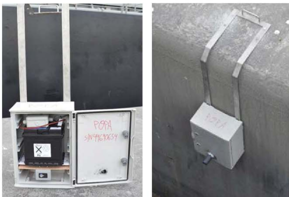
Figure 6. LDM and installation over the dock wall.
