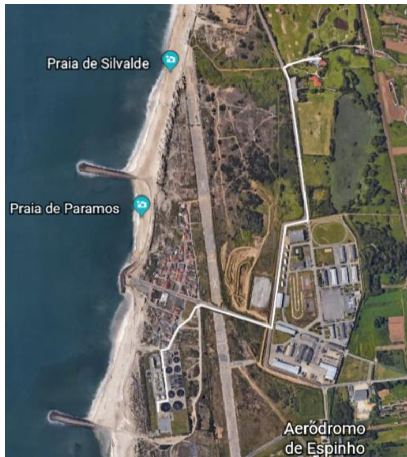
Reclaimed water pipeline (in white) from the WWTP to the Golf course
