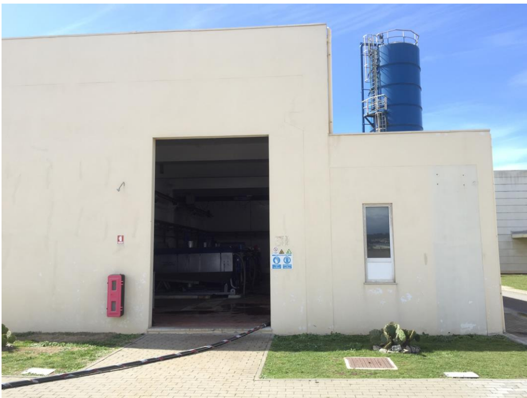
Dewatering/mechanical thickening facility
