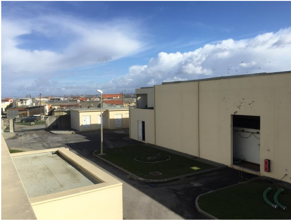
Preliminary treatment facility
