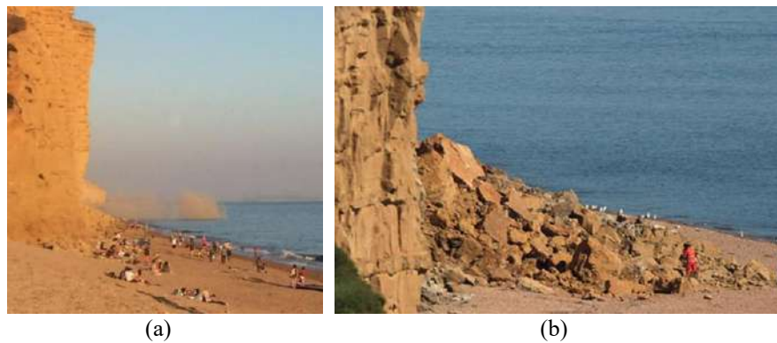
Fig. 2. Cliff collapse: (a) stones falling on bathers [5]; (b) emergency services searching the rubble [6].
