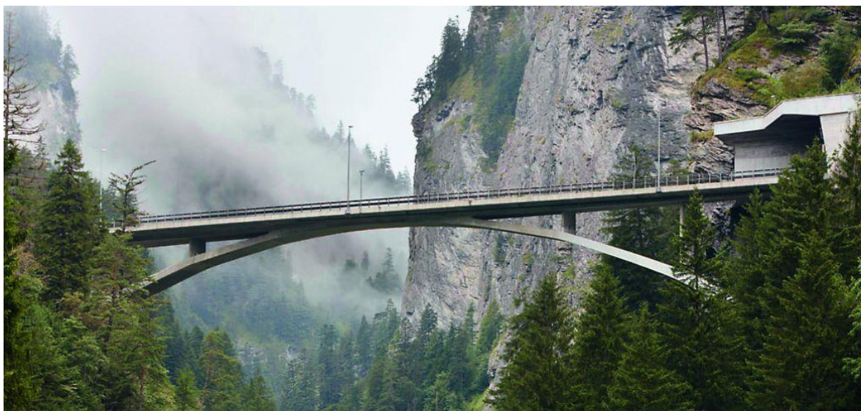
Figure 3: Viamala Bridge in Thusis (Switzerland) by Christian Menn
