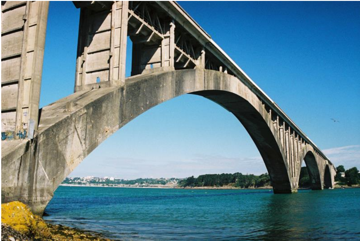
Figure 13: Pont Albert Louppe, Plougastel by Eugene Freyssinet
