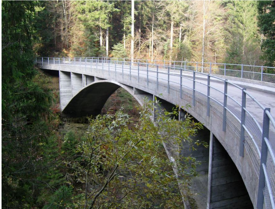
Figure 2: Schwandbach Bridge by Maillart
