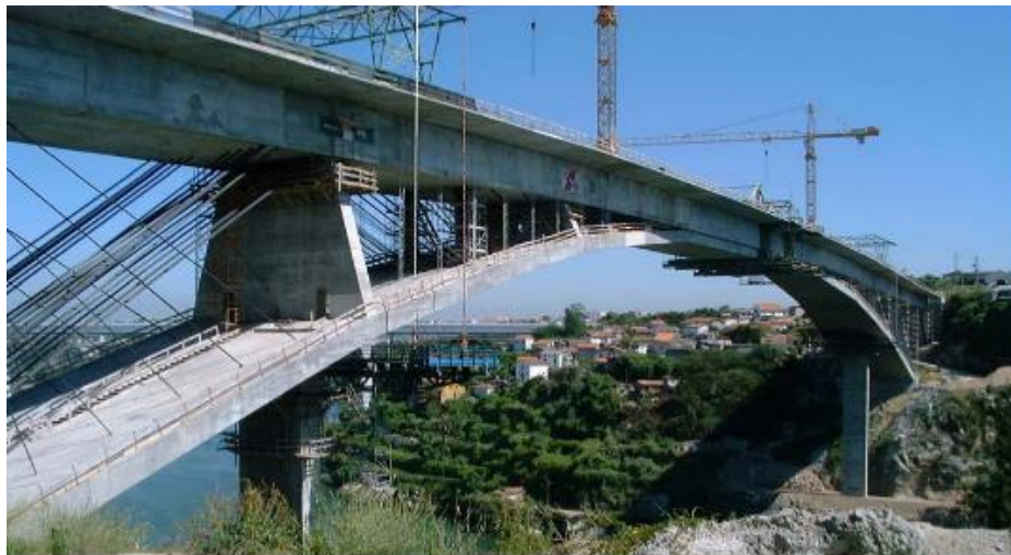
Figure 10: Finished construction before removing the temporary stability elements
