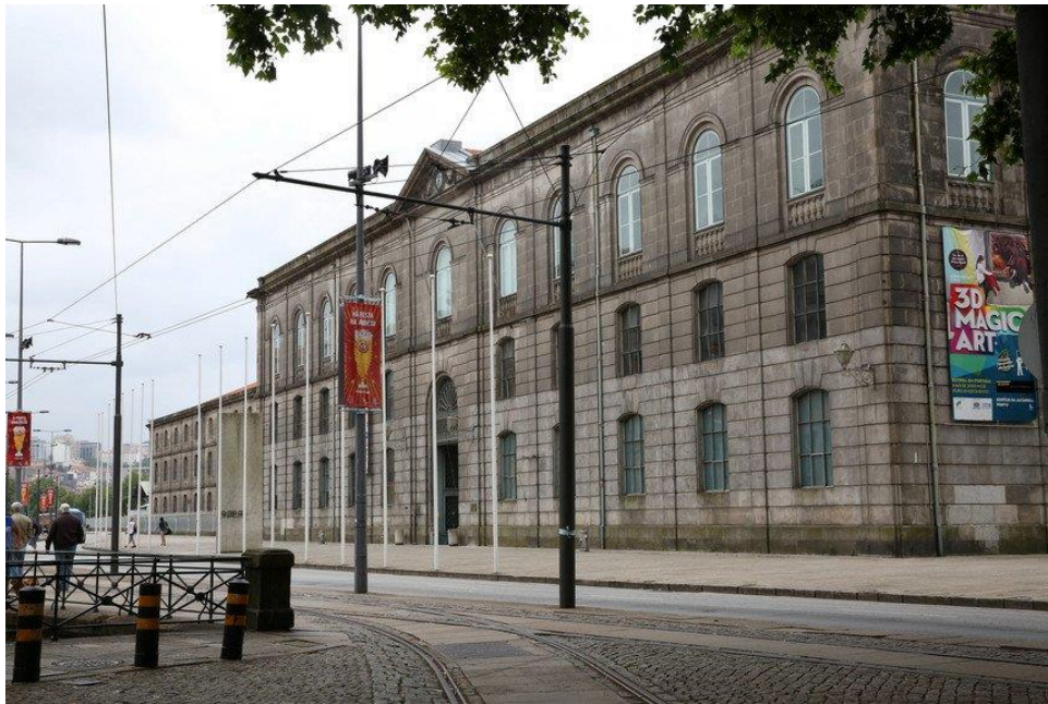
Figure 29 "Rua Nova da Alfândega" and the building "Alfândega Nova"
