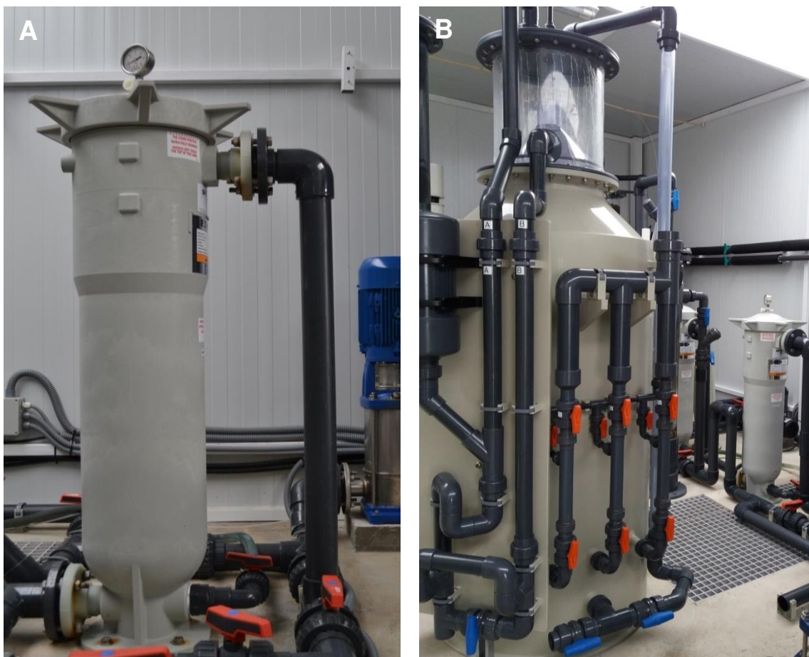
Fig. 8 – Equipment used at RiaSearch for solid waste removal, including a housing unit with a bag filter inside (A) and the protein skimmer (B). Photography courtesy of Adriana Laranjeira, RiaSearch.
