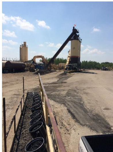
Figure 2-14. Sampling asphalt materials from different plants in Illinois
