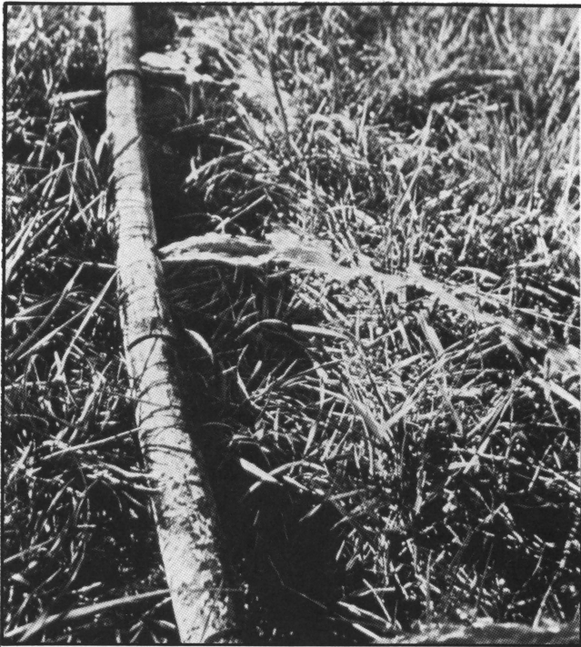
Figure 1. Plastic pipe with properly spaced holes may be suitable for small lagoons.
