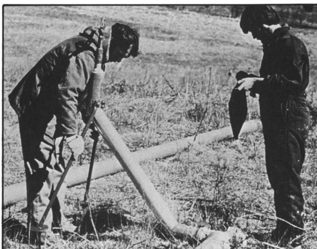
Figure 5. Hand-set sprinklers are placed at proper intervals along the main line.
