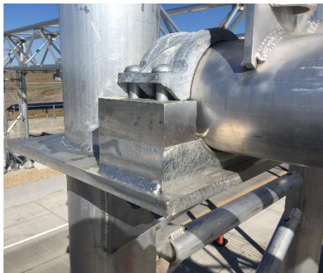
(a) Connection for Bottom Chord
