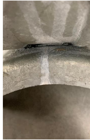
(b) Crack on the Other Side Propagated to the Edge
