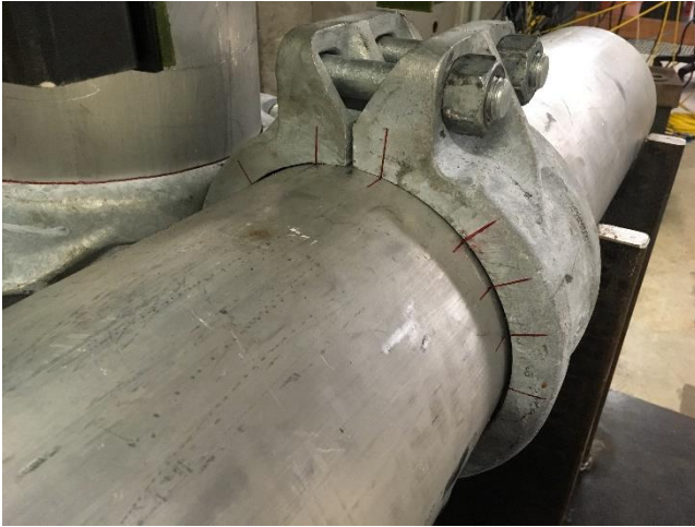
(a) Markers on Horizontal Pipe
