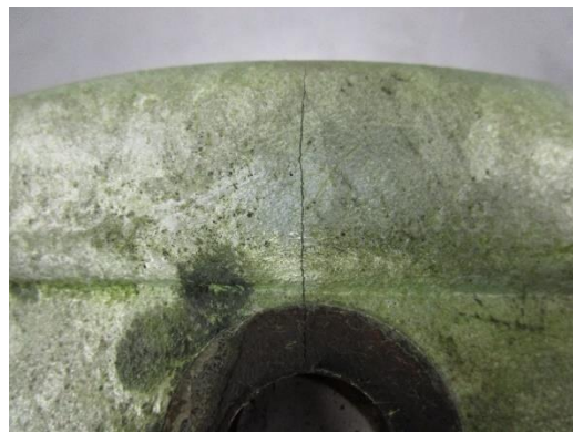
(b) Crack on the 10-in. Coupler
