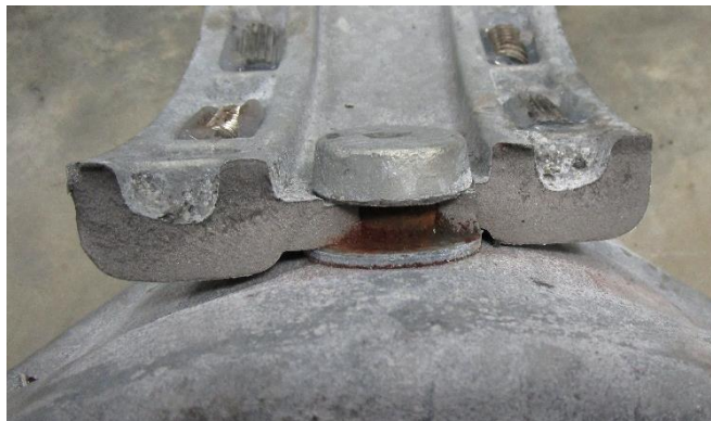
Figure 47. Corrosion Products on Failure Surface of FAT-TENS4
