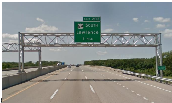
Figure 1. Bridge-Type Overhead Truss Sign Structure (OHTSS)
