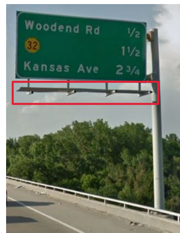
Figure 4 Steel grate walkway on a two-chord COSS
