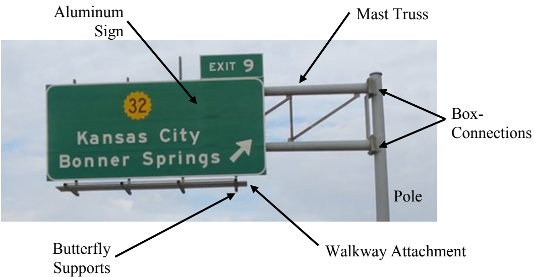
Figure 12 Constructed KDOT COSS
