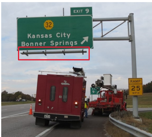
Figure 3 Steel grate walkway on a two-chord COSS
