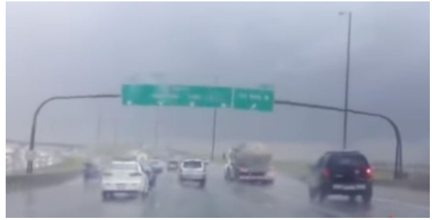
Figure 10 Monotube OSS experiencing galloping effects of vortex shedding (upward) (Mangat 2016)
