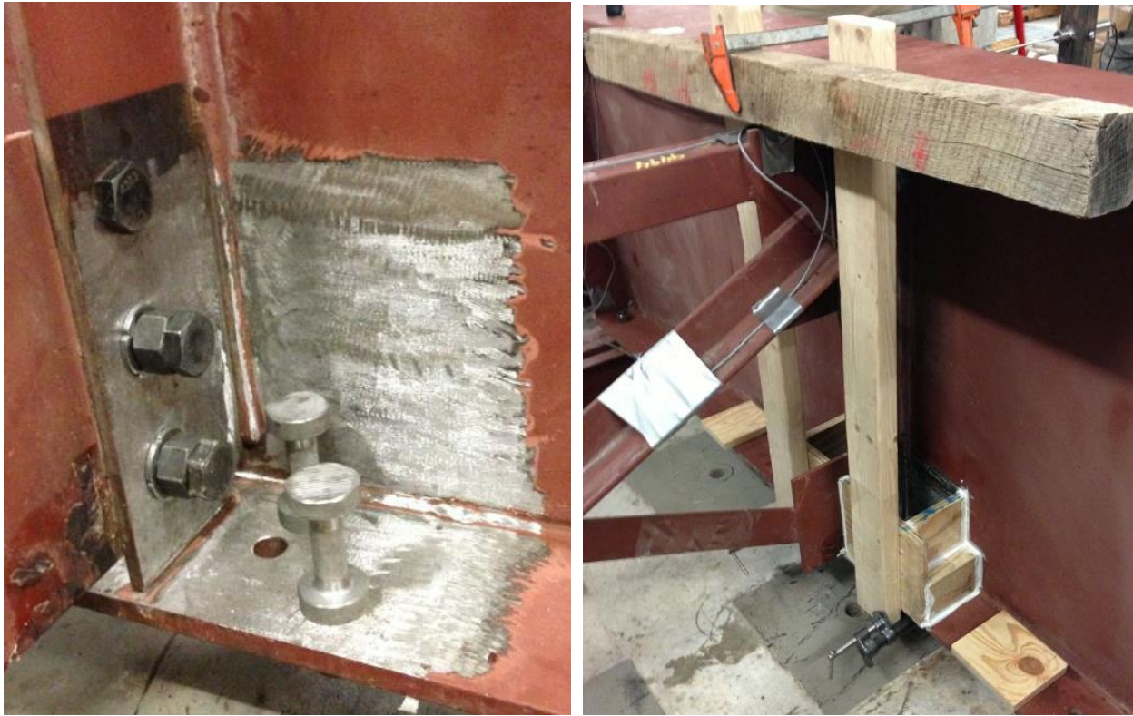
Figure B 3: Web-gap region prepared for the composite block retrofit
