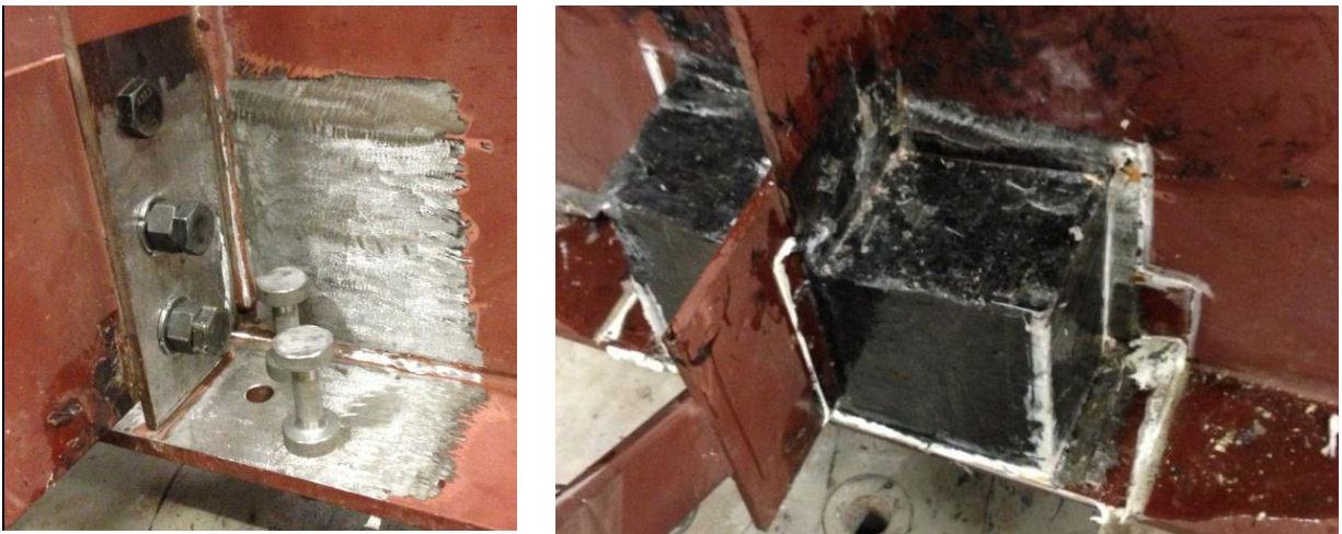
Figure 4 Repair for girder subassembly 2 prior to and after casting CFRP block.
