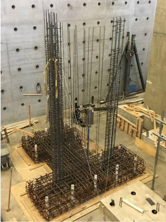
(a) Base block steel cage
