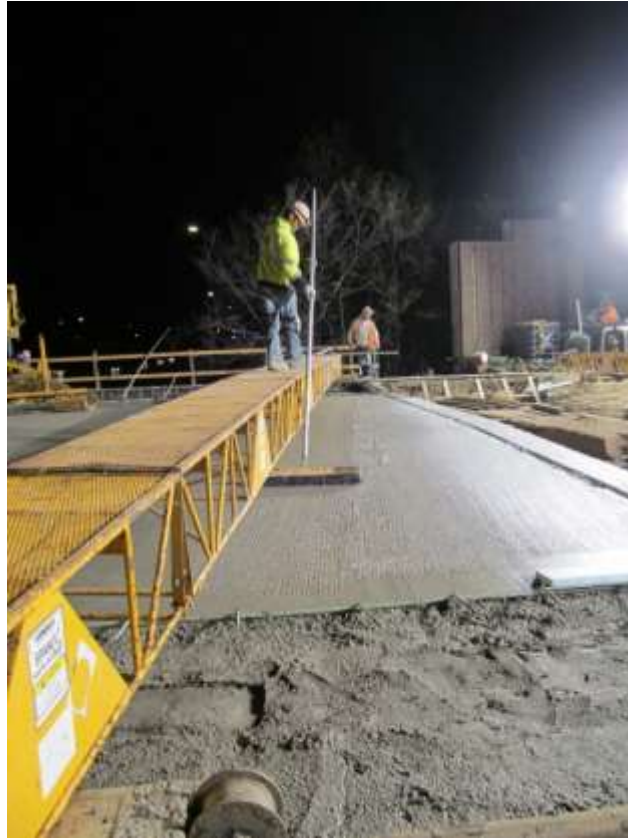
Figure 4.9: IC-LC-HPC-4 Tining and unfinished sidewalk section
