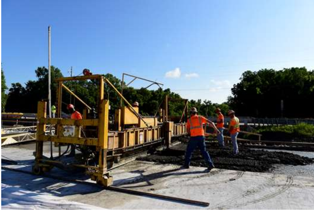
(a) Overlay concrete placement
