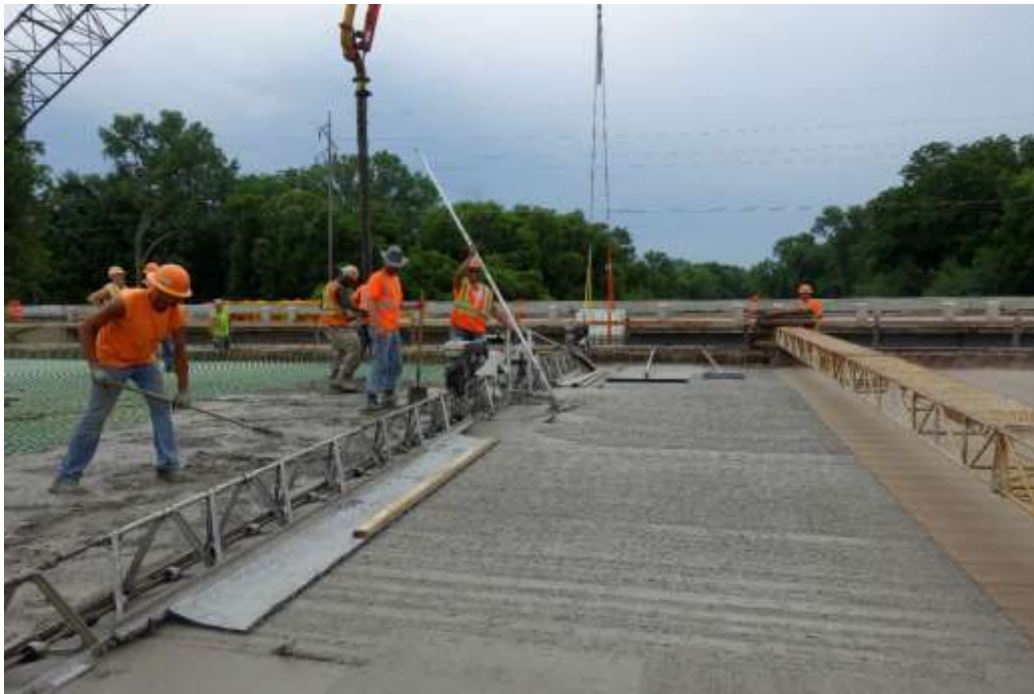
Figure 4.4: Placement, finishing, and curing setup for IC-LC-HPC-2
