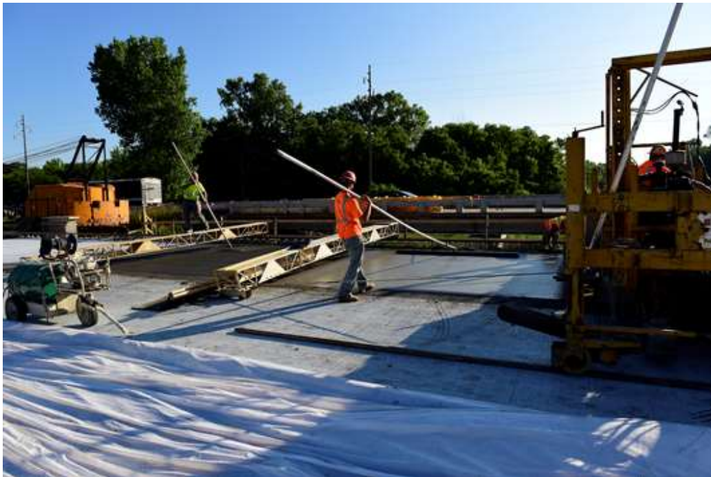
(b) Overlay concrete finishing
