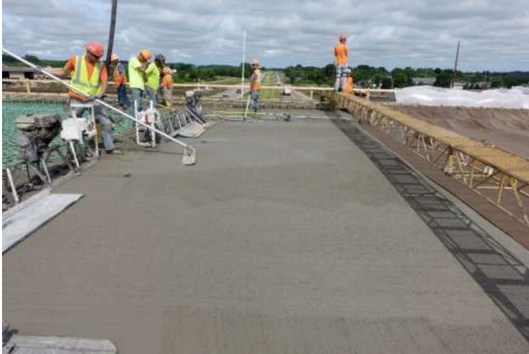
Figure 4.7: Placement, finishing, and curing setup for IC-LC-HPC-3
