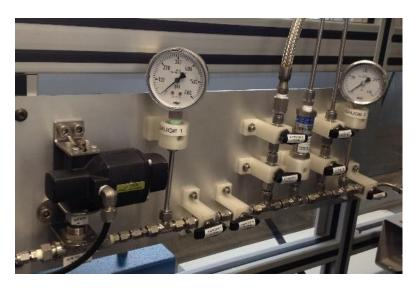
**Figure 7.2.** Pressure Gas Panel that houses the pressure gauges, Air-to-Open Valve, and vent lines
