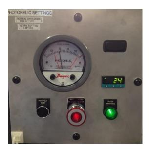
Figure 7.1. Photohelic Unit with Emergency Crush Button
