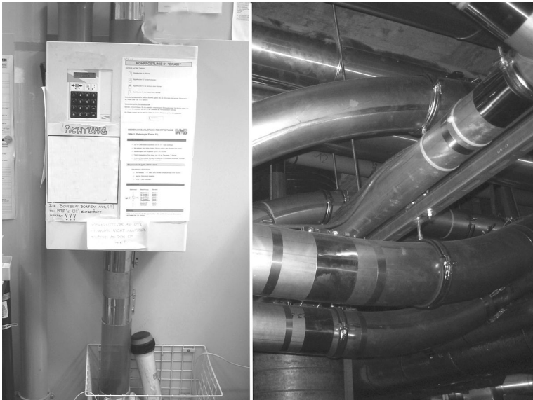
Figure 3. Hospital system for pneumotransportation of materials between different units; transport of urgent biopsy to Pathology Department.
