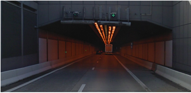
Fig. 1. Entrance of the Beveren Tunnel in Antwerp
