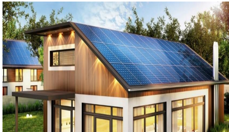
Fig. 39: Solar panels example
