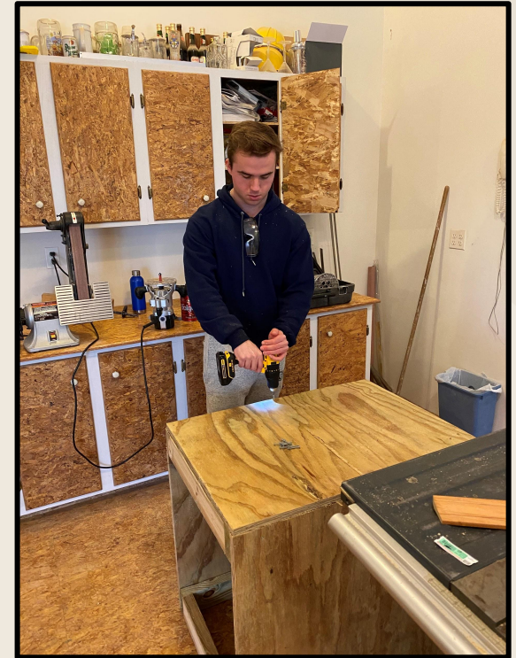
Nick Cauley Working on Cabinet Build
