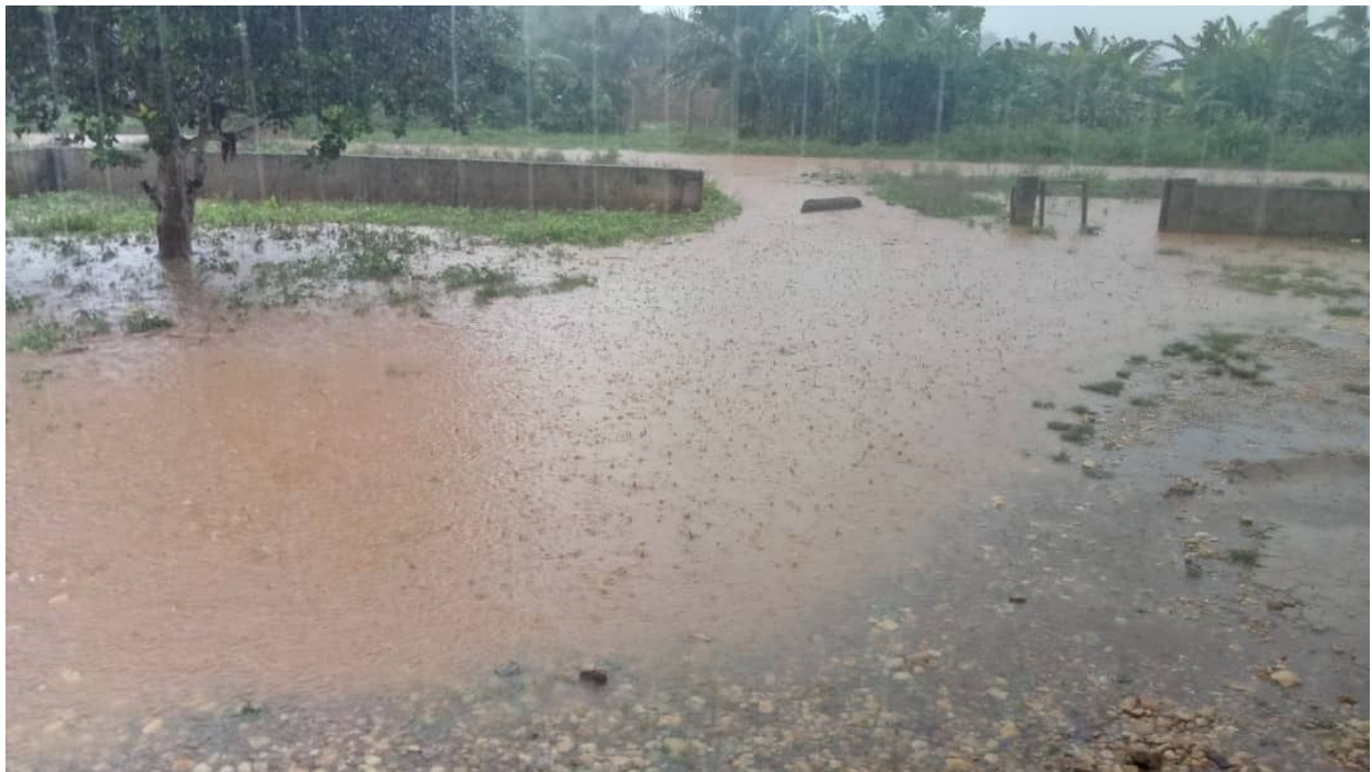
Figure 4: Road runoff flooding the parking lot (Photo Credit: Gloria, Director of the Health Center).
