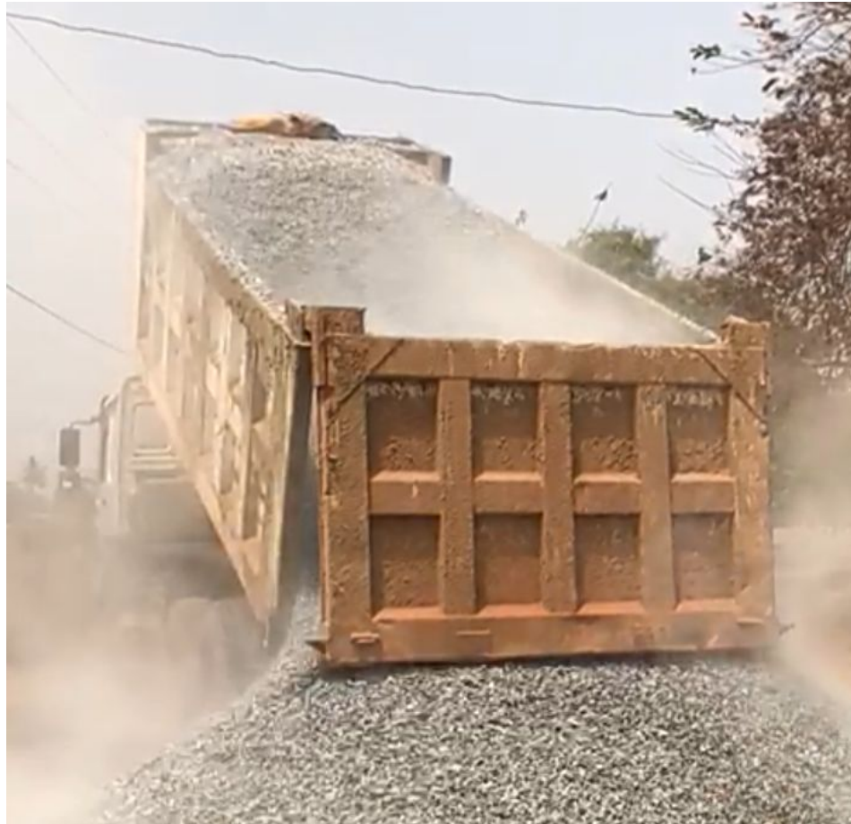
Figure 8: The gravel being delivered on the 16th of February, 2020
