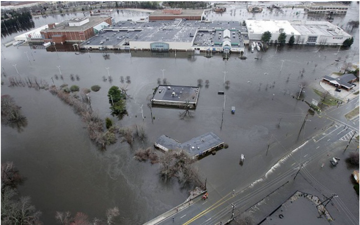
FIGURE 3 Flooding of Warwick Mall (in the Main Branch of Pawtuxet River) during March 2010 event (credit A. P.)
