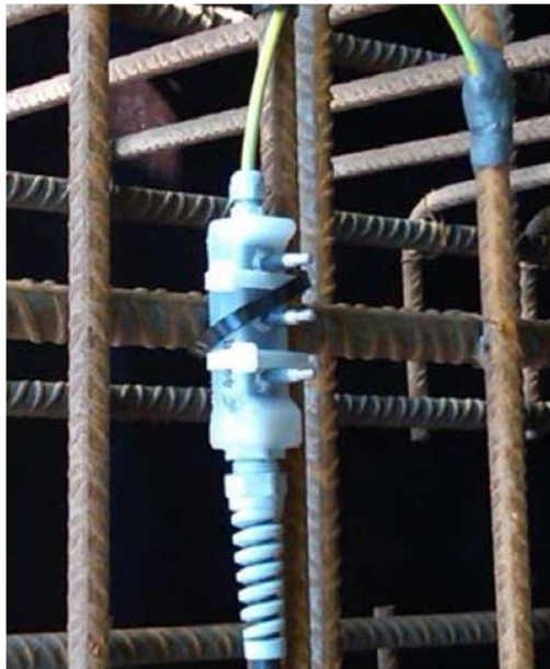
Figure 2-39: Installed M3 probe prior to placement of concrete [36]
