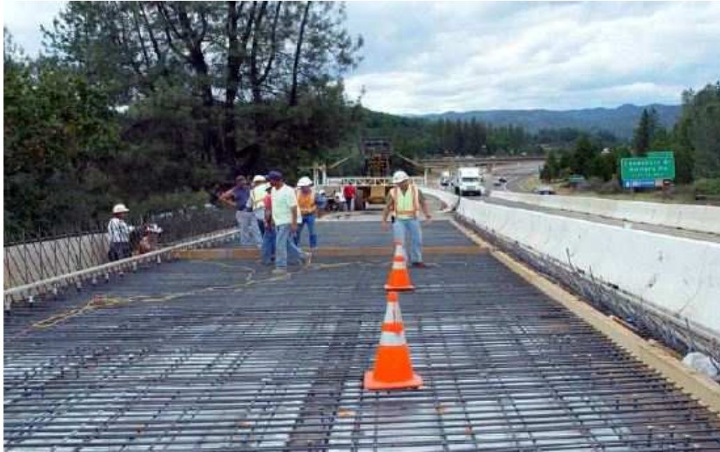
Figure 2-18: Placement of ECI-1 units prior to concrete placement [23]
