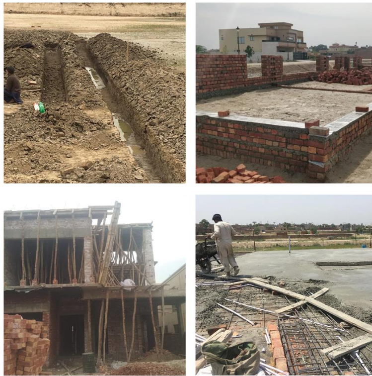
Figure 30 (Typical residential construction site in Lahore. Image Source: Surblund Consultants, Lahore)
