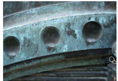
Figure 1r. Copper1: Close-up detail of decorative copper geometrically designed, architectural detail with significant blue-colored patina.
