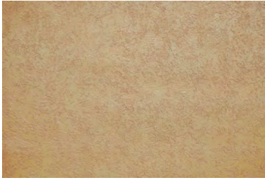
Figure 1y. Stucco3: New stucco wall with smooth, regular features.
