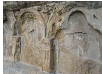
Figure 1i. Stone2: Close-up of carved sandstone (face-bedded) wall with significant surface detail loss due to erosion.
