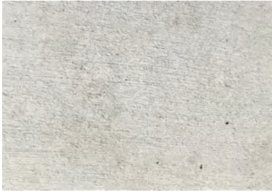
Figure 1m. Concrete3: Close-up of new concrete wall with regular, smooth surface.
