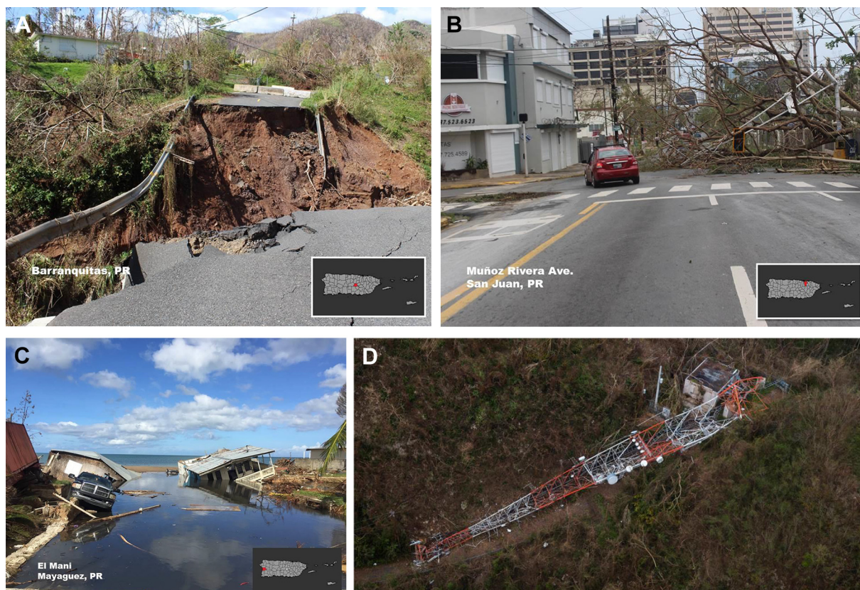
Figure 4 Representative photos of damage from Hurricane Maria (A–C). 24 Of the 1600 cellular antenna towers in Puerto Rico, only 15% to 20% continued to operate after Hurricane Maria (D). Photo: Archivo/GFR Media. 25
