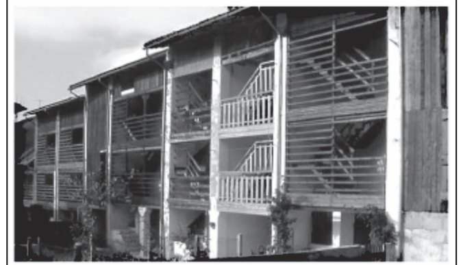
Figure 6 - Above: evolutionary and aggregative scheme of Andreis houses. Below: rustic, mono and bicellular buildings, alternate in the continuity of the andreane ranks (Chinellato et al., 2002).
