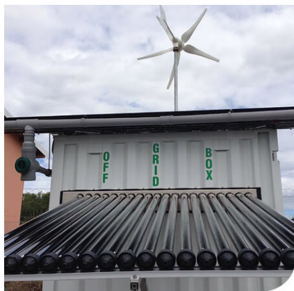
Figure 30: OffGrid Box container with a wind turbine
