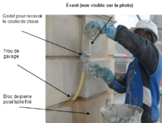
Figure 20- Grout injection
