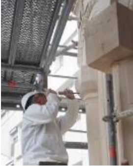
Figure 4- Stone cutting – Colombes church
