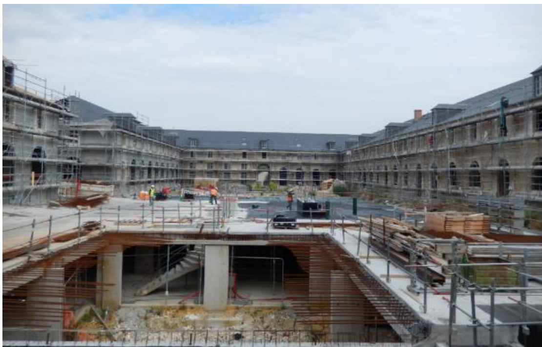
Figure 26- Work in progress - Compiègne
