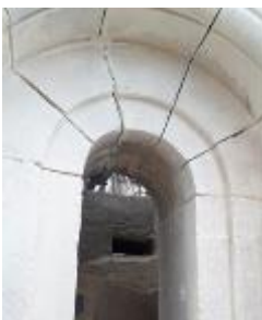
Figure 6- Example of an arch segment
