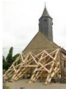
Figure 16- Buttress shoring and shrinking
