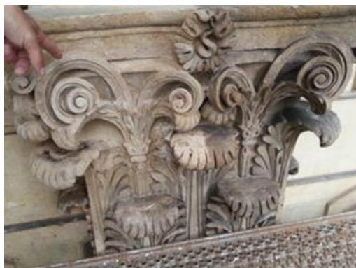
Figure 19- Example of cleaning facing – Madeleine Church
