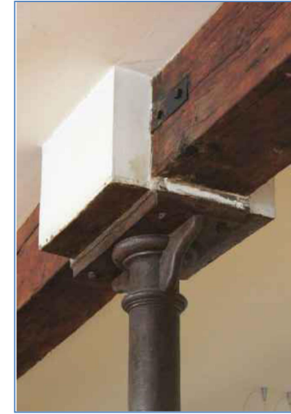
1st FLOOR - Columns
