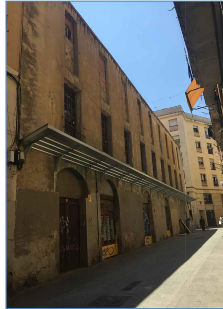
GUIFRE FACADE -Facade arches
