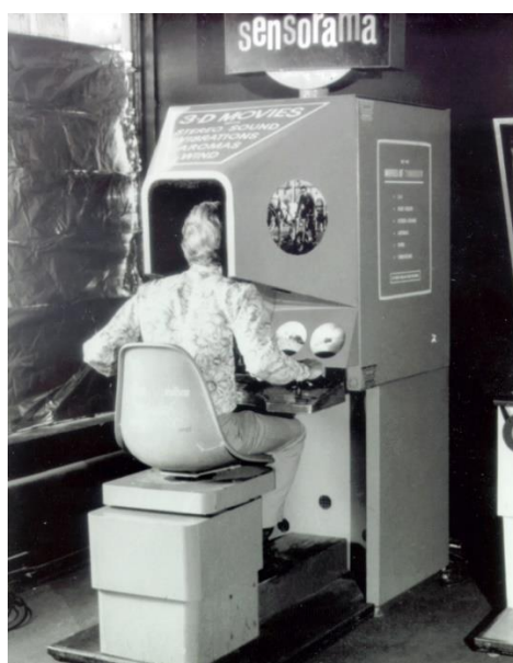
Figure 3.2 The Sensorama VR machine.
