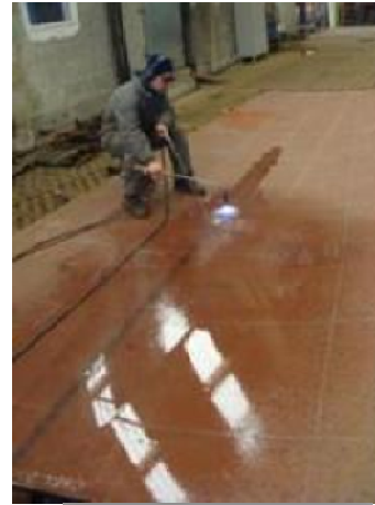
Figure 1: Manual line Heating forming
