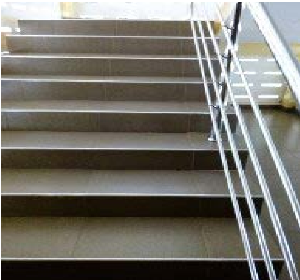
Figure 6.2: Stairs with handrails at the new administration block in PUC
