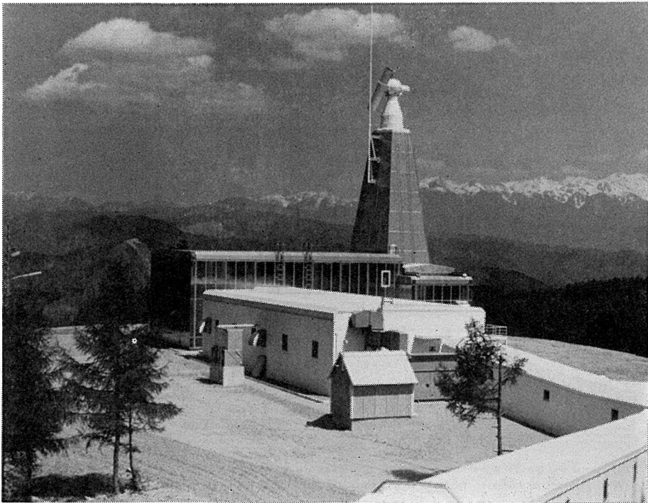
Fig. 5. General view of the Domeless Solar Tower Telescope to the East. The tower is covered with temperature controlled stainless panels. Besides the upper six stages, buildings are covered with mere stainless steel plates. Neighboring building and passage-way are coated with titan-white paint.
