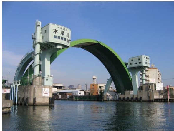
Fig.3 Visior gate in a river mouth ( presented by Osaka Prefecture)
