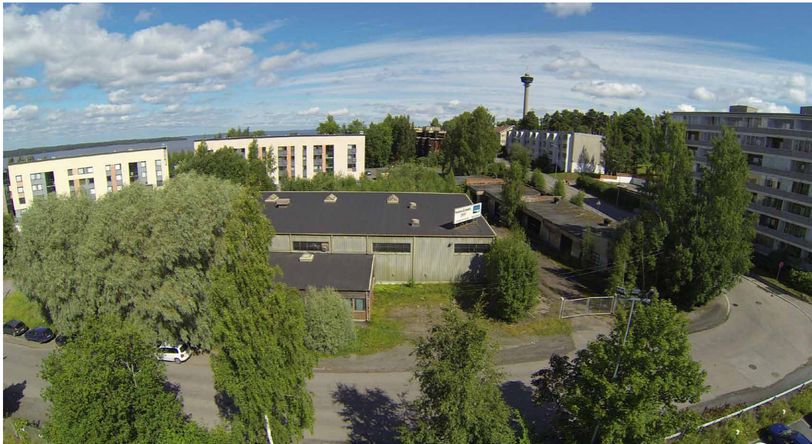
Picture 3.3. The three buildings in the middle of the picture in Onkiniemi will be pulled down due to traffic arrangements. Source: Rantatunneli Alliance
