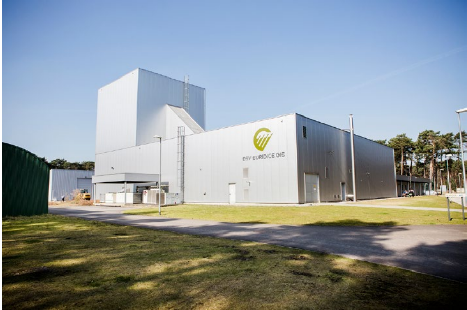
Figure 4. The building hosting HADES shaft 2.
