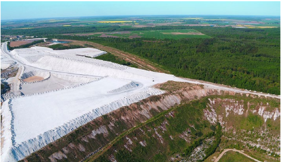
Figure 33. A typical pile of phosphogypsum, which is a common NORM.
