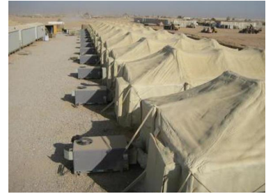
Figure 5: 36,000 BTU/hr environmental control unit (left). ECUs externally installed in support of insulated fabric tents (right), from [48] and [49].
