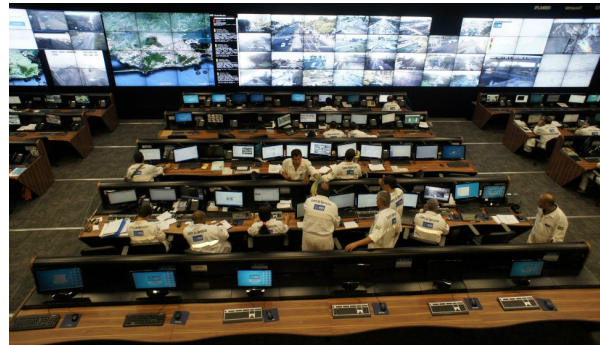
Joint Operations Center
