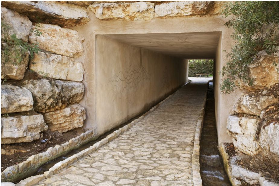
Figure 8: View of the Entrance Tunnels after their restoration, October 2008. Photo by J. Galanti.
