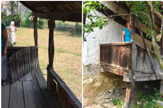
Figure 7: Porch on the southeast side of the house
