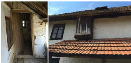
Figure 8: Left - A handy pantry next to the entrance porch on the northwest side of the house; Right - Abdestana (niche for ritual washing) upstairs (above the entrance porch on the southeast side of the house)
