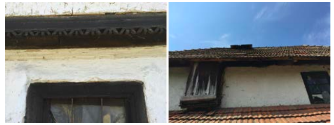
Figure 9: Left - Ground floor cantilever transition is further emphasized by a decorative, profiled plank; Right - Smoke vent (badge) from the garret space to the open space
