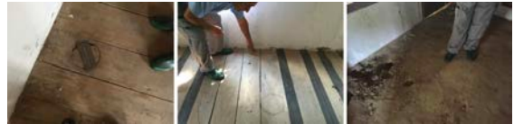
Figure 27: Left - A lid in the floor through which hot air was introduced from the ground floor room where the furnace was burning; Middle - The opening in the floor from where the cable went to the front door to the house - the "remote control" system; Right - Ground floor in the "house" ("kuća") area
