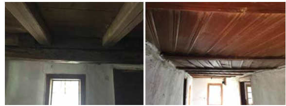
Figure 20: Left - Ground floor-first floor structure above one part of the "house" ("kuća") space; Right - Wooden ceiling ("šiše") in divanhana space
