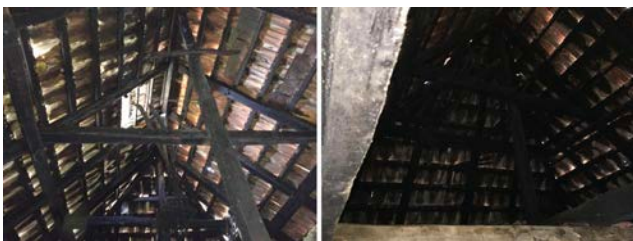
Figure 19: Roof construction (see wooden grate-shelf for drying cheese)
